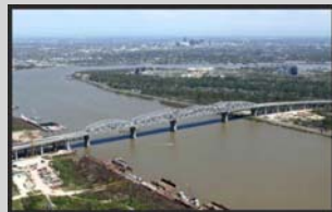
HPL Bridge was expanded to 3 wider lanes in each direction
